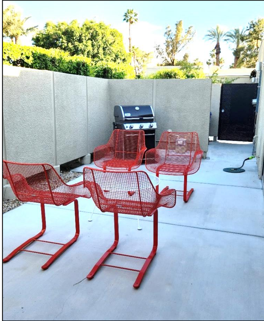
Inside the east patio looking SSE. Note the footings elevate the patio wall to provide air circulation and visual "lightness."
