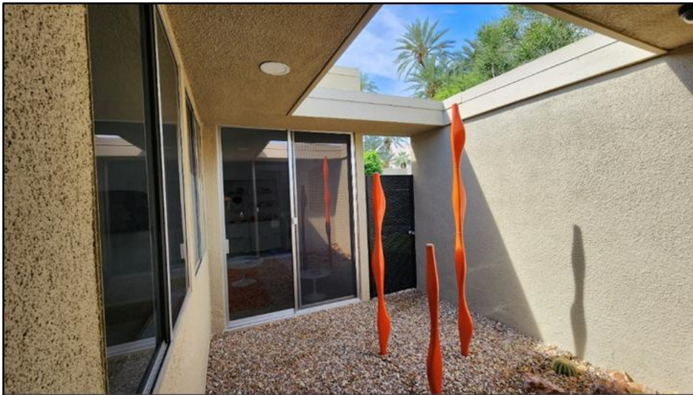
The west atrium remains intact and features generous eaves on three sides, aluminum-framed horizontal sliding windows (left), and aluminum-framed sliding glass doors. This view also shows the lower (thicker) and higher (thinner) cornice and metal drip-edge flashing details. This view is through the sliding glass doors on the north side of the atrium looking SSW.
