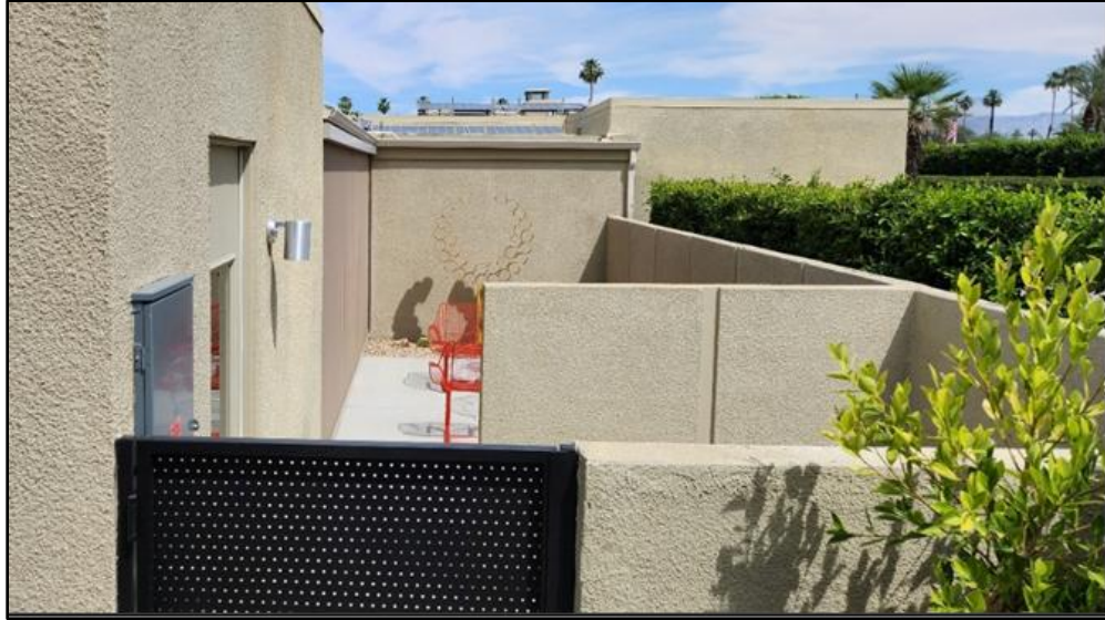
The original walled east patio showing a later (but early) extension (foreground). Also seen is the perforated metal gate, electrical panel, kitchen door, cylindrical lighting fixture and sliding glass doors (covered with retractable shade in this photograph). This view is from south looking due north.
