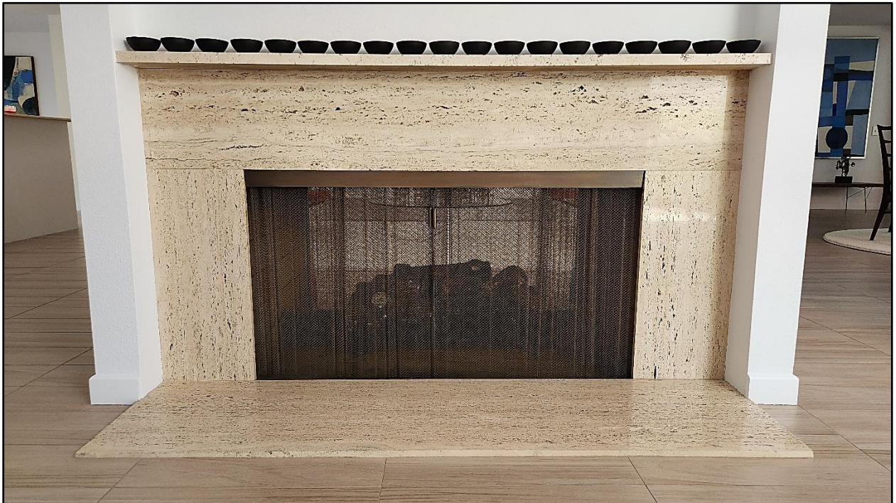
A notable extant interior architectural feature of Tamarisk Gardens #5 is the double-sided (or “see-through”) fireplace surrounded by travertine stone.
