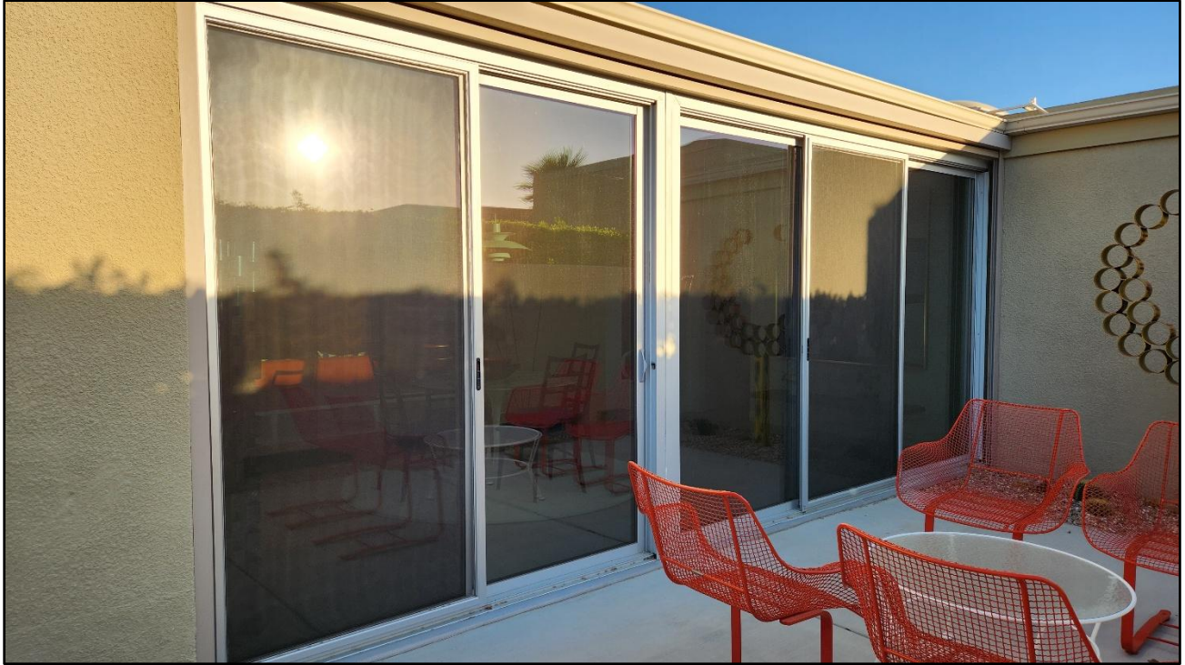
Looking NW from the east patio, these sliding glass doors (installed prior to 1973) turned the original garden room into interior space.
