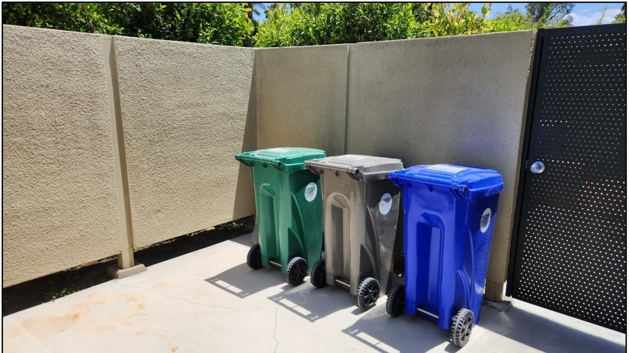
Looking SE into the east patio's trash enclosure. This wall extension was added prior to 1973 and is comparable to the original build in quality of workmanship. However, it can be distinguished by its square concrete footings (as opposed to the cylindrical concrete footings used in the original build).
