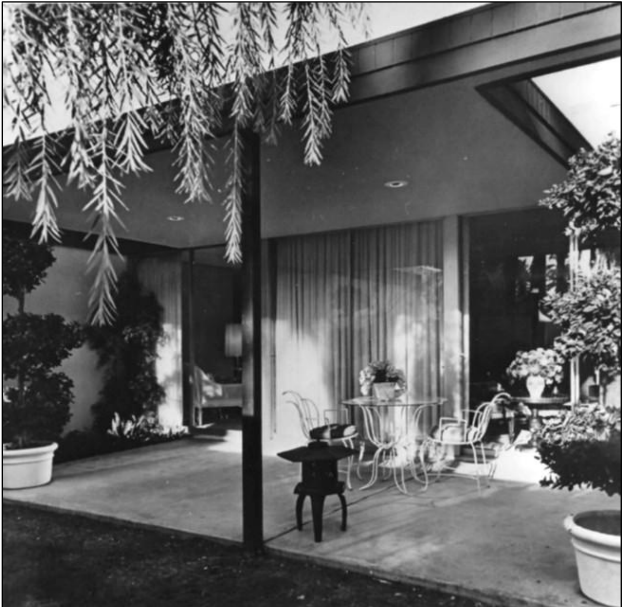
Shown here is a circa 1965 publicity photograph of a Tamarisk Gardens “garden room.” Note that a structural roof, with electrical service, is already in place. Throughout Tamarisk Gardens, this space was closed in and the small open-air gap (seen at upper right) was covered with a skylight.
