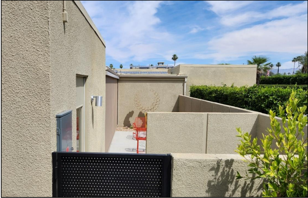
Looking due north over the patio gate into the east patio.
